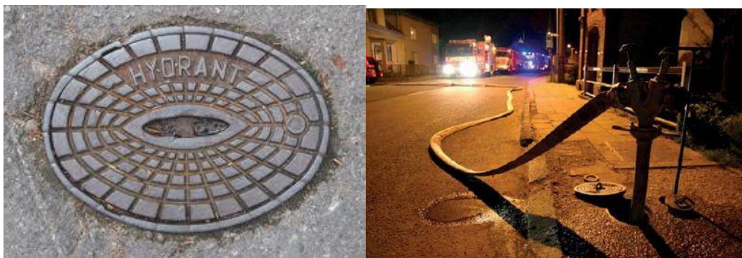
Fig. 12. Underground hydrant and its usage
