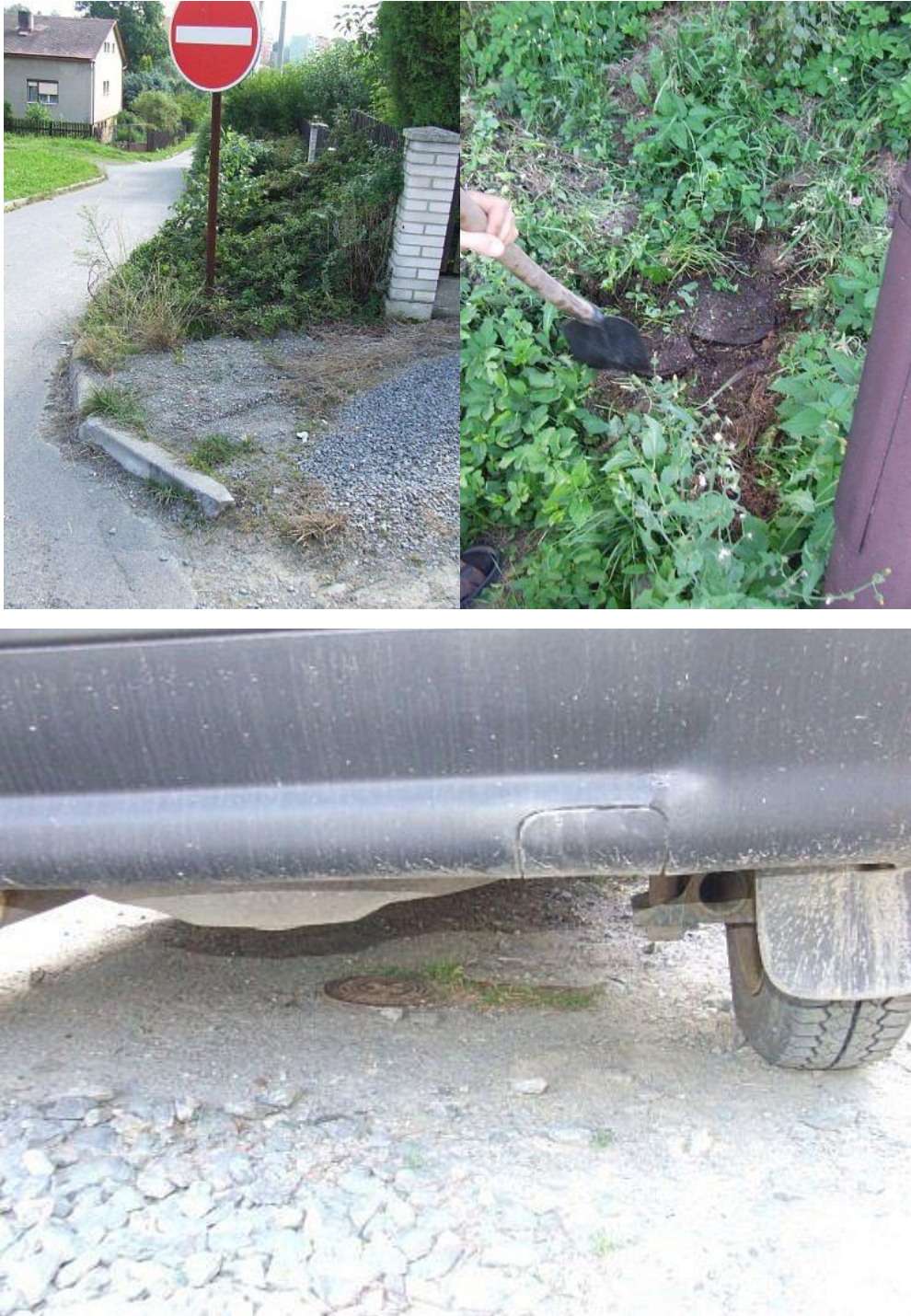
Fig. 19. Limited access to underground hydrants (Kúdela, 2010)
