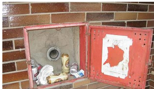
Fig. 25. Inappropriate use of dry riser in building (Křečková, 2010)
