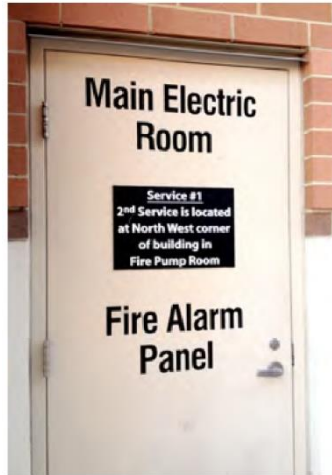
Fig. 10. A room with signage indicating (top to bottom), the main electric service, the location of a secondary electric service, and the fire alarm system control panel. (OSHA, 2015)
